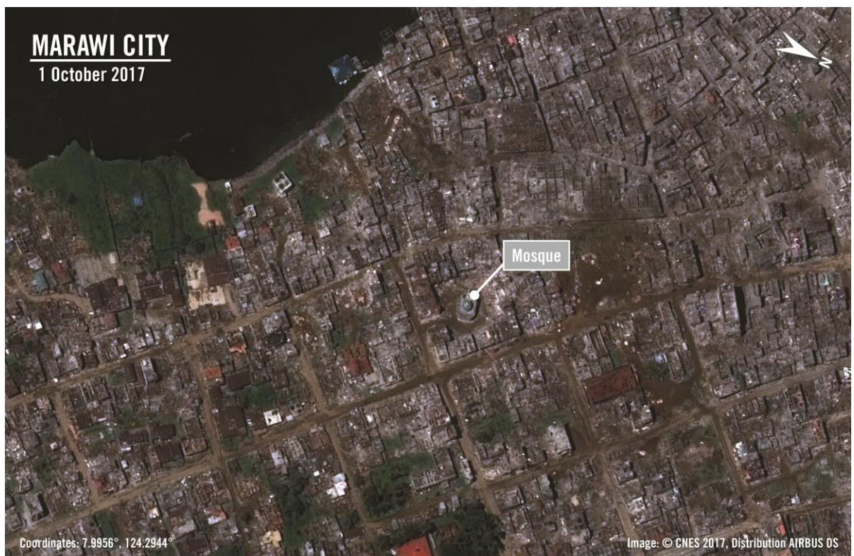
A closer look at the main battle area in eastern Marawi as seen in the lower satellite image from 1 October 2017 shows the area almost completely destroyed, compared to what it looked like in the upper image from 31 January 2017 before the fighting began.
