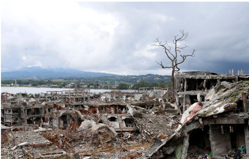
Mangled structures are seen in the main battle area in Marawi city, shown to the media during a tour by the military, 25 October 2017. © Jeffrey Maitem/Anadolu Agency/Getty Images
