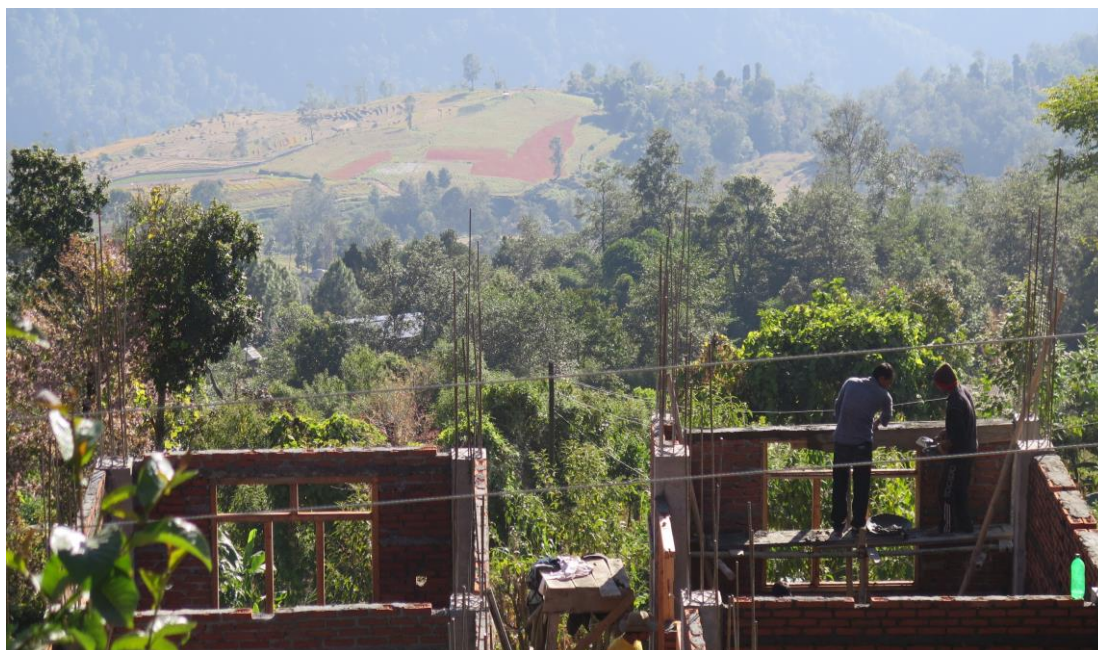
Rebuilding a house in Khabre VDC, Dolakha District, November 2016. © Amnesty International
