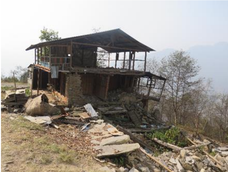
A house destroyed in the 2015 earthquakes in Dolakha district, Nepal. © Amnesty International
